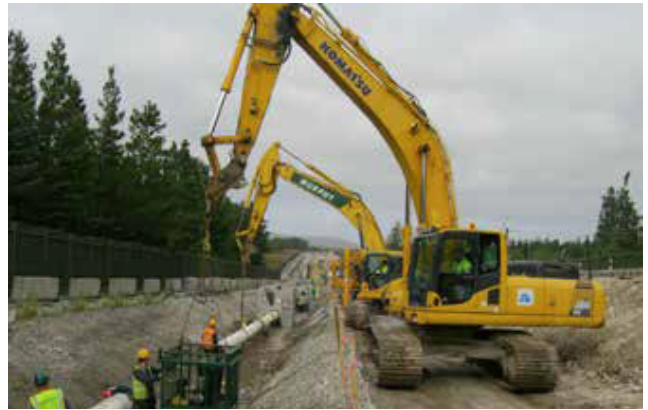
Figure 5. Welding on spread.
