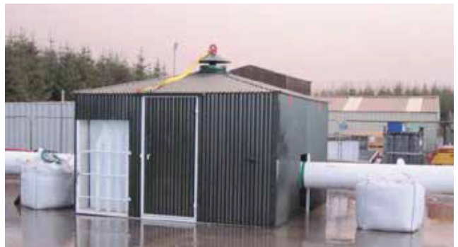
Figure 6. Improved welders habitat.
