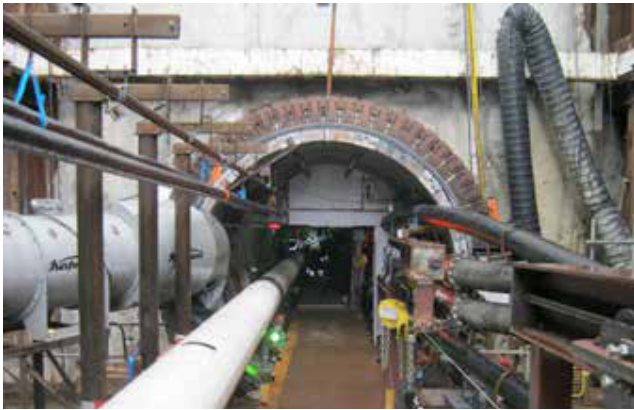
Figure 4. Gas pipe entering tunnel.
