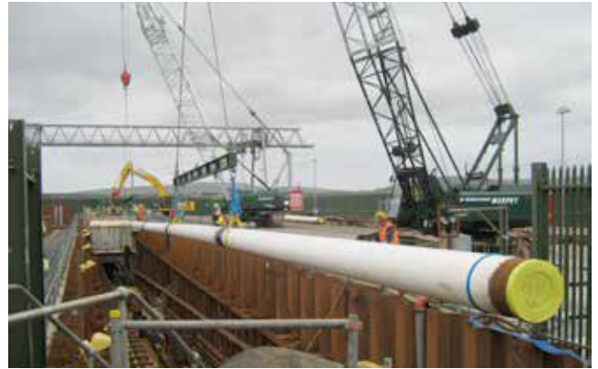
Figure 3. Gas pipe lowered into pit.
