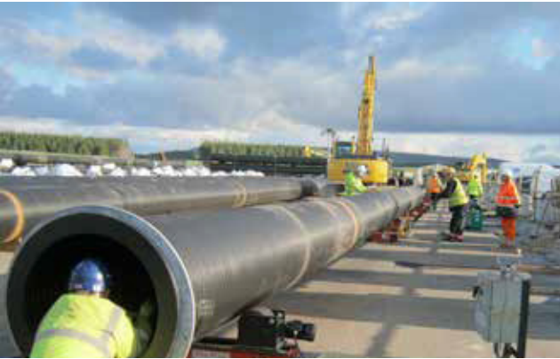
Figure 2. Assembling vent pipe strings in the yard.
