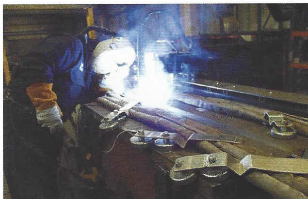
Figure 1. Welding of 50mm plate.
